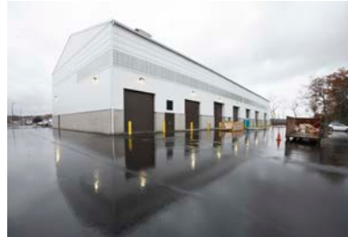
Rocky Hill Repair Facility
