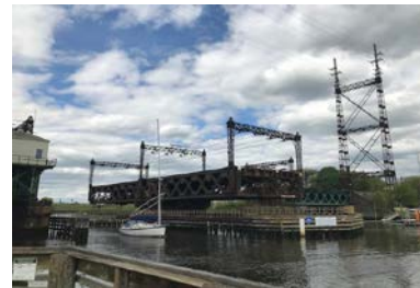
Walk Bridge Program
