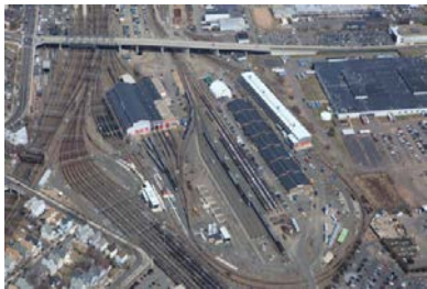
New Haven Rail Yard Master Complex
