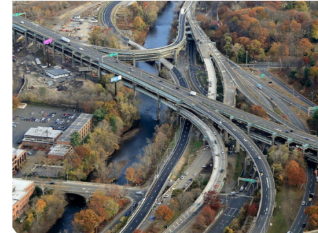
I-84 / Route 8 Waterbury Mixmaster Rehabilitation
