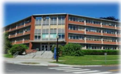
Monteith Building Renovation
